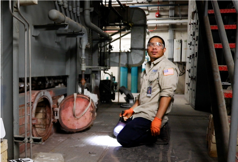
Central Plant Operator Shyreal Salogaol cleans one of UCR's boilers by crawling through a circular door opening in preparation for the annual inspection. (UCR/Erin Chapman)
